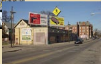
A new square is proposed on a vacated gas station site.
