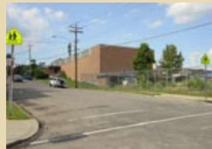
The existing Rockdale School building will be demolished to make way for a park.
