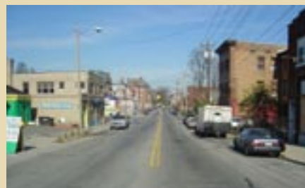
Burnet Avenue—Many abandoned buildings and vacant lots about the street.
